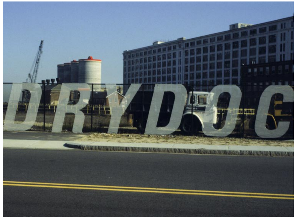
Below: Taking advantage of a common element on the site, chain-link fencing, entrance and dry dock identification signs are constructed of 8' high white chain-link letters mounted on existing fencing.
