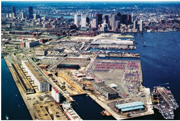
Above: Boston's Marine Industrial Park was developed on the site of an old military base and includes a diverse mix of tenants, including the Massport Cruise Terminal, the Boston Design Center, light manufacturing, and fishing and shipbuilding industries. In part, the intent of the signage and graphics program was to help provide a unifying element throughout the site.
